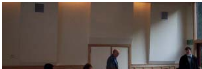
A finished wall...
